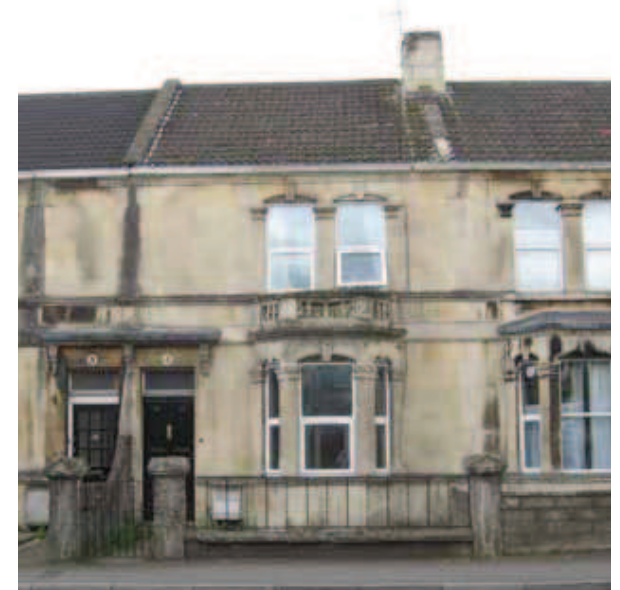
Example of a Victorian/Edwardian Building in Bath & North East Somerset
