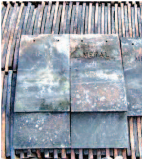
Responsibly sourced used materials eg. reusing roof tiles
