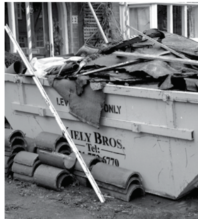
Segregating waste onsite for recycling
