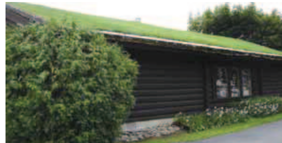
Green roofs can help reduce pollution and surface water run-off and are particularly useful in dense urban areas.
